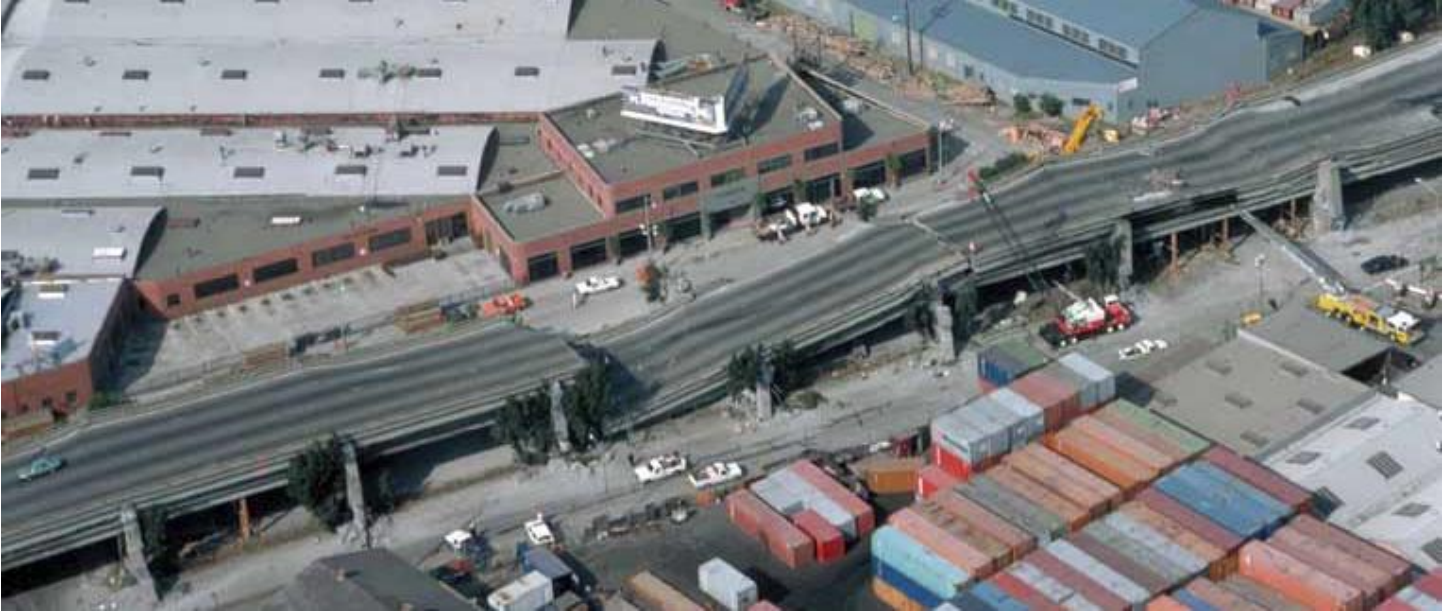
Collapsed section of ramp to the Bay Bridge in San Francisco, CA
